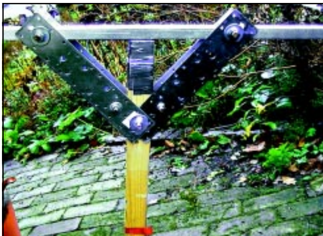
Temporary plates for the boom-to-sub mast.
