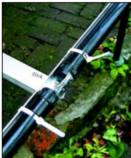
The antenna elements secured to the angle sections.
